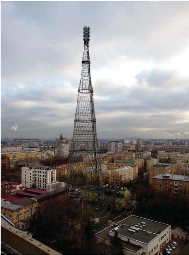
Fig. 1. Shukhov tower in Shabolovka, Moscow, general view.
