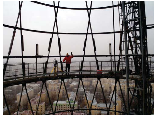
Fig. 2. Laser scanning at the 100-m level.
