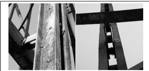
Fig. 3. Fastening of the 1st intermediate ring of the 1st section to a leg through a U-shaped bracket.
