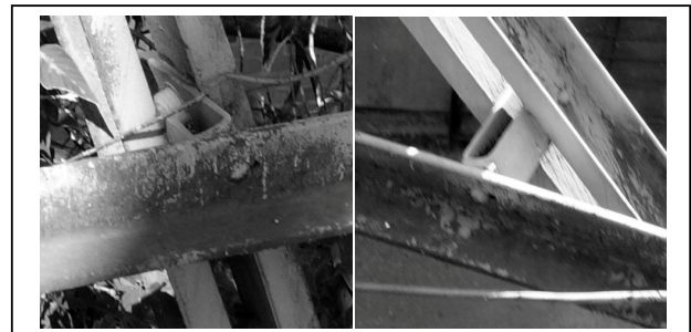
Fig. 5. Unused holes in the 2nd intermediate ring of the 1st section.
